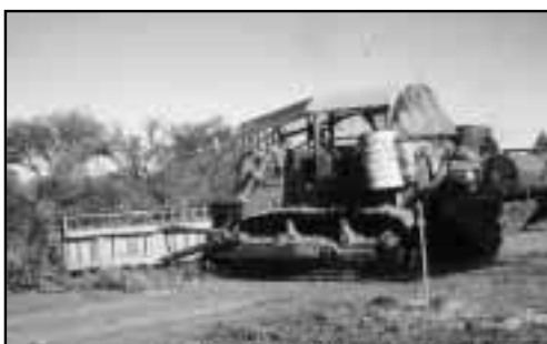
Bulldozer clearing prickly acacia
